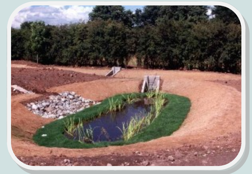
Spillage basin newly constructed (Bob Bray)
